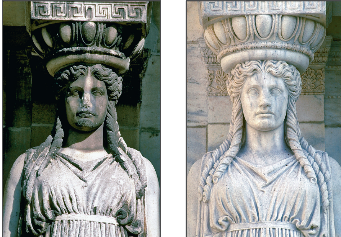
FIGURE 16.13B A statue in Chicago damaged by acid rain, before (left) and after (right) restoration.
